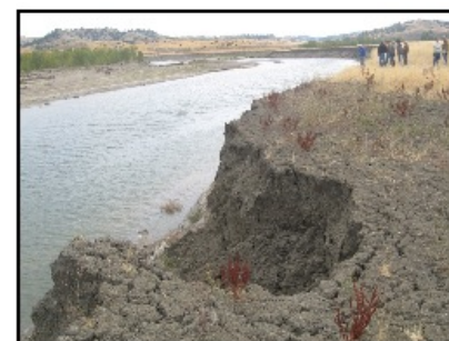
Figure 6. View upstream of eroded pump site showing ongoing failure of high bank.
