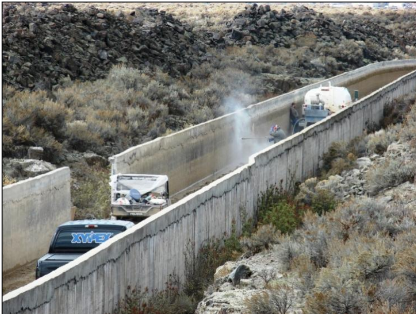
Milner-Gooding Canal – rehabilitating concrete channel near Shoshone November 11, 2015
